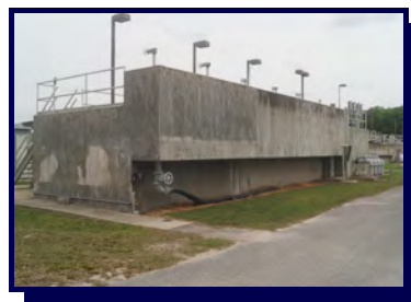
CCC Sump and CCC No. 1
