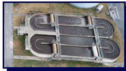
Lakeside Oxidation Ditches
