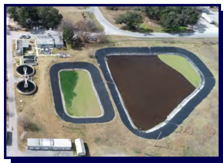
Reject Water Storage Ponds
