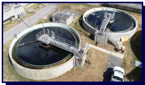
Secondary Clarifiers (50-foot diameter)
