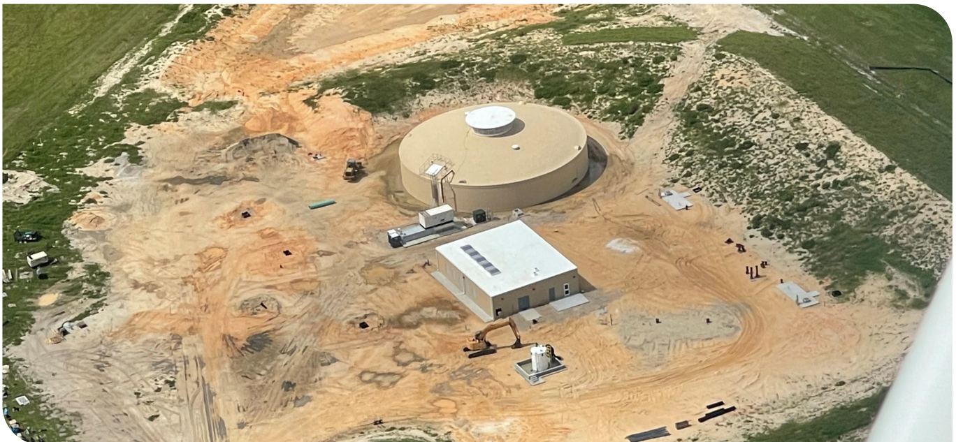
Pictured is an aerial of the construction of the Gibson Place Utility Water Treatment Plant to serve The Villages. This design-build project was fast-tracked due to the rapid growth of the area. Halff provided water plant design, permitting, and construction administration services.
