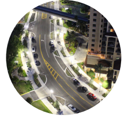
Riverplace Boulevard Complete Street Jacksonville, FL
