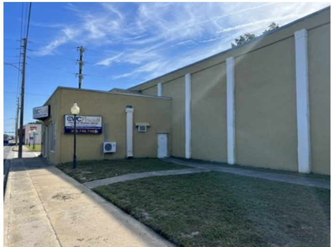
Exterior View of Subject
