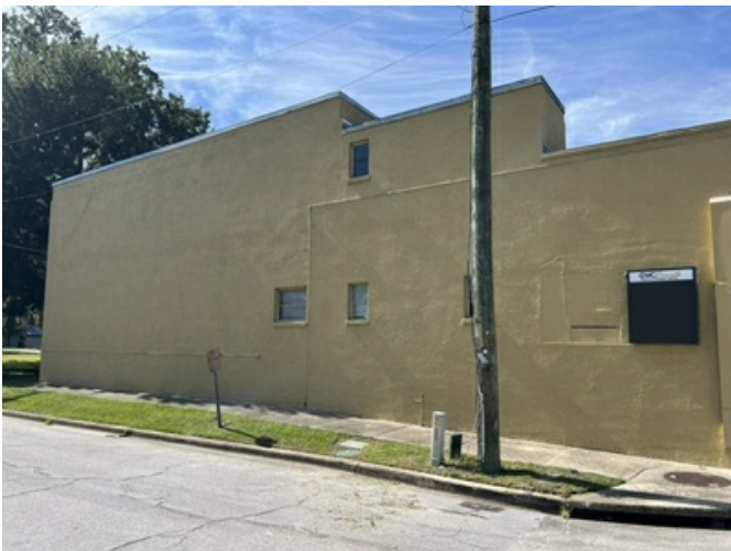
Exterior View of subject
