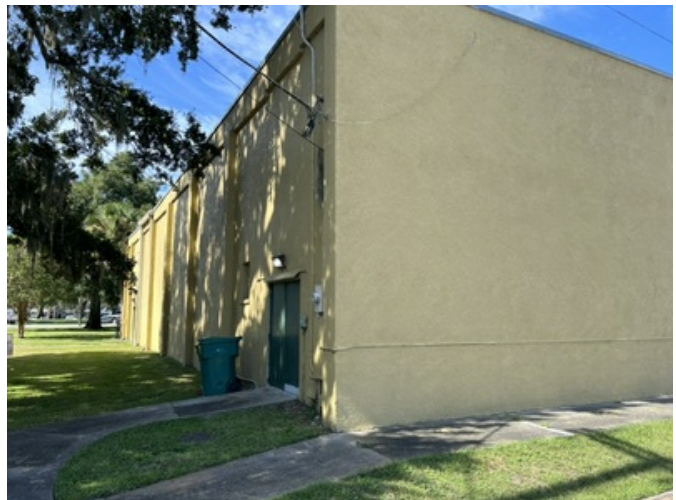
Exterior View of Subject
