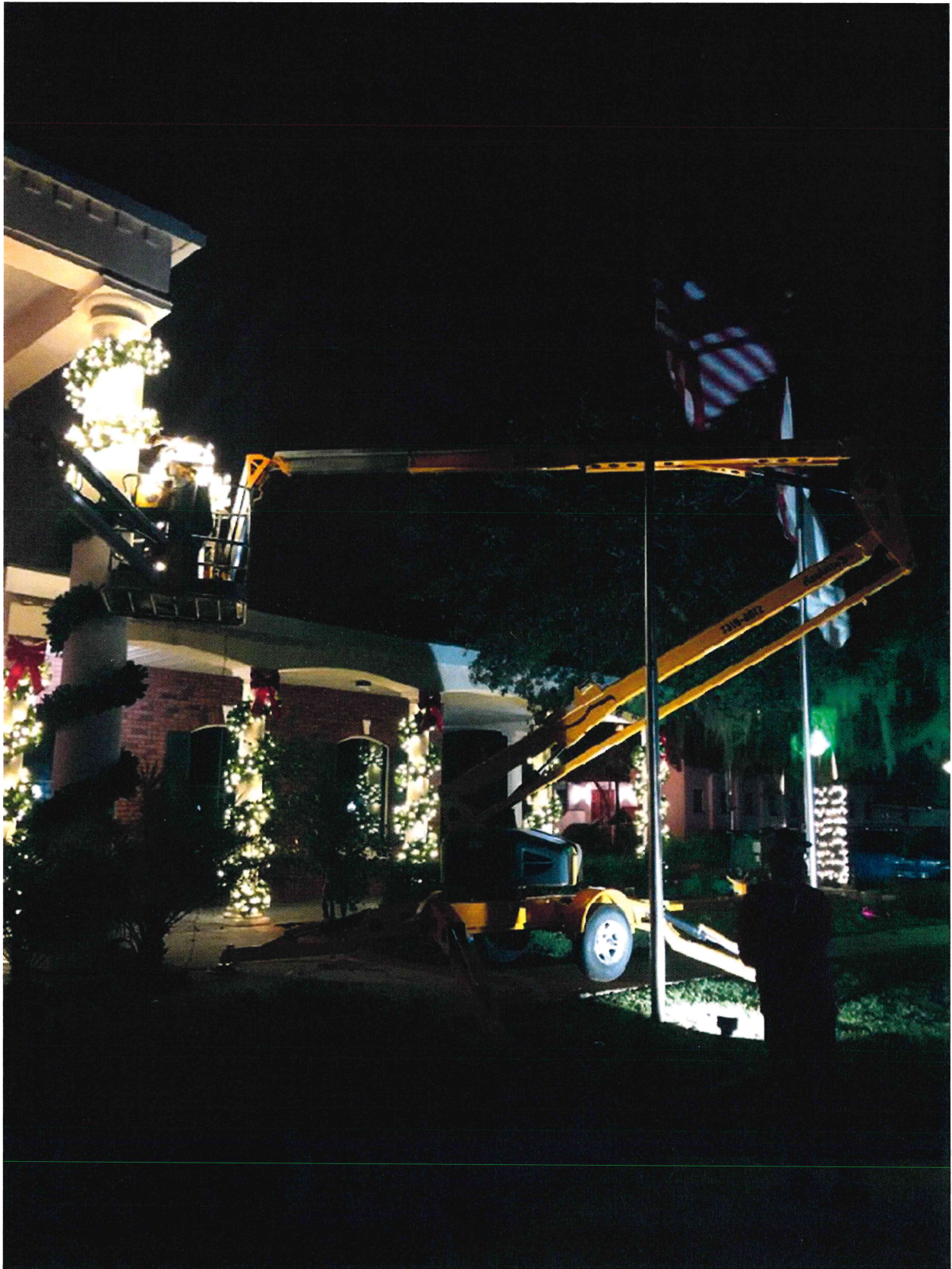
Installation of lighted Garland on City Hall. Done after hours to prevent interruption of city business.
