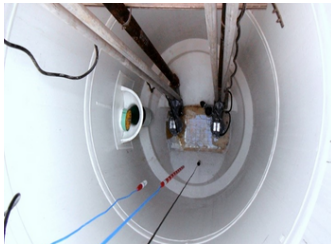
Wet well coating pic
