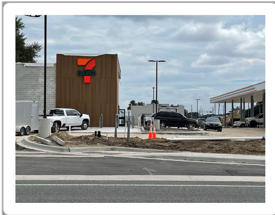
7-Eleven Convenience Store/Gas Located at the corner of US 301 and CR 472
