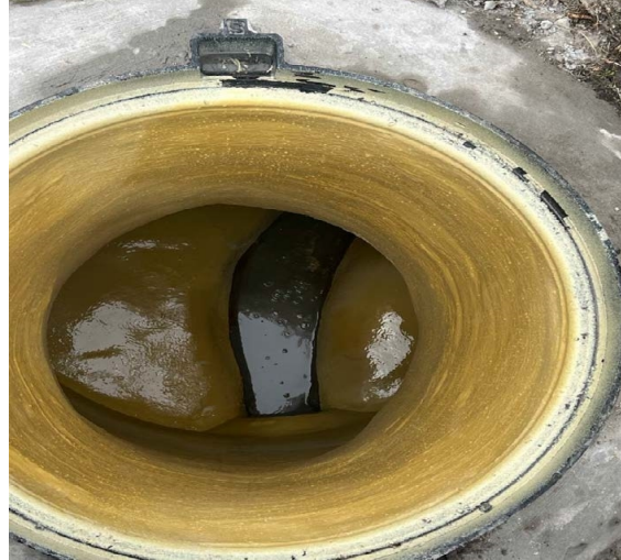
MANHOLE REHAB WITH EPOXY COATING
