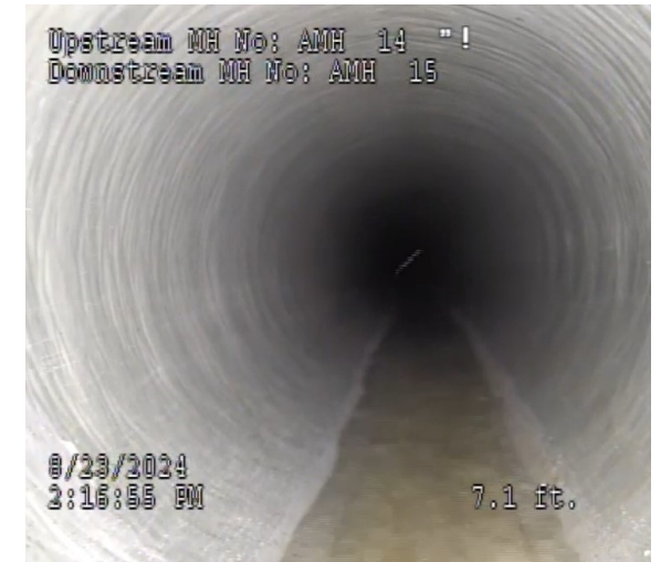
NEW LINED IN PLACE REPAIR OF DAMAGED GRAVITY MAIN
