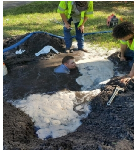
LIVE MAIN LINE REPAIR IN CONTINENTAL
