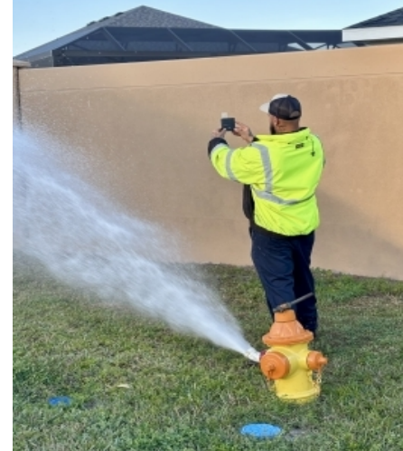
DEAD END AND MAIN LINE FLUSHING
