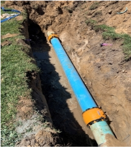
12" WATER MAIN REPAIR IN OXFORD OAKS
