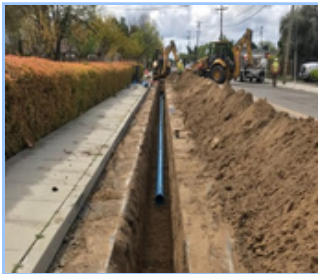
Water Main Pic
