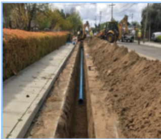
Water Main Pic
