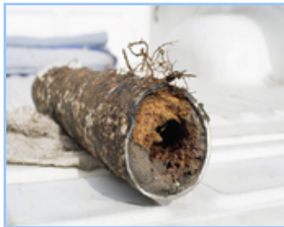
Sewer Main Repair
