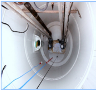
Wet Well Coating Pic
