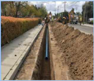
Water Main Pic
