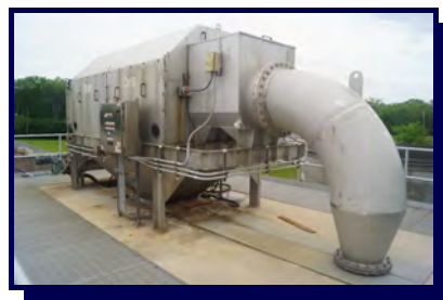
Mechanical Drum Screen
